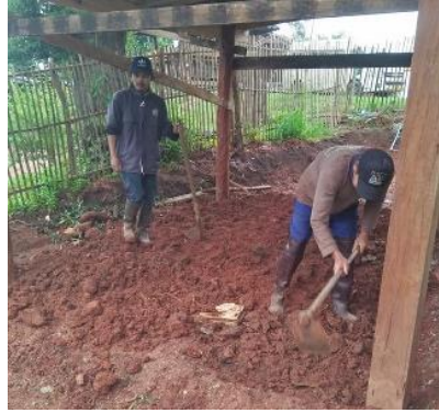
The kitchen building work
